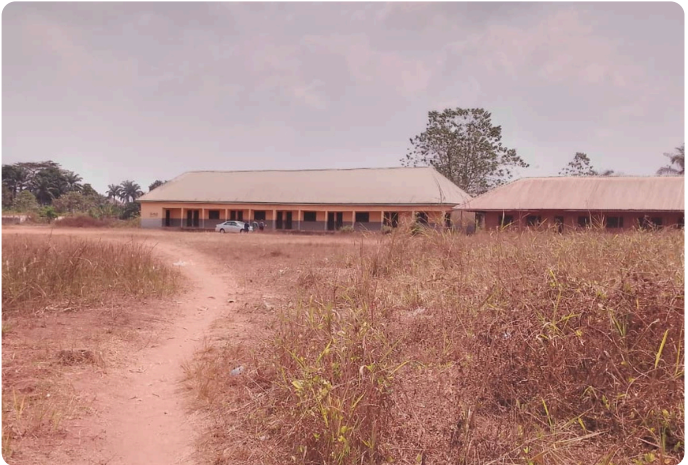
Our new playground construction site, provided by Obodo Village with the authority of the Ikeduru Local Government Council
